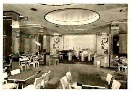
The glass-walled Glass Hat at the Belmont Plaza presented extreme acoustic difficulties which were overcome by velocity microphones. The speaker units with directional baffles are concealed behind grilles in the walls.
